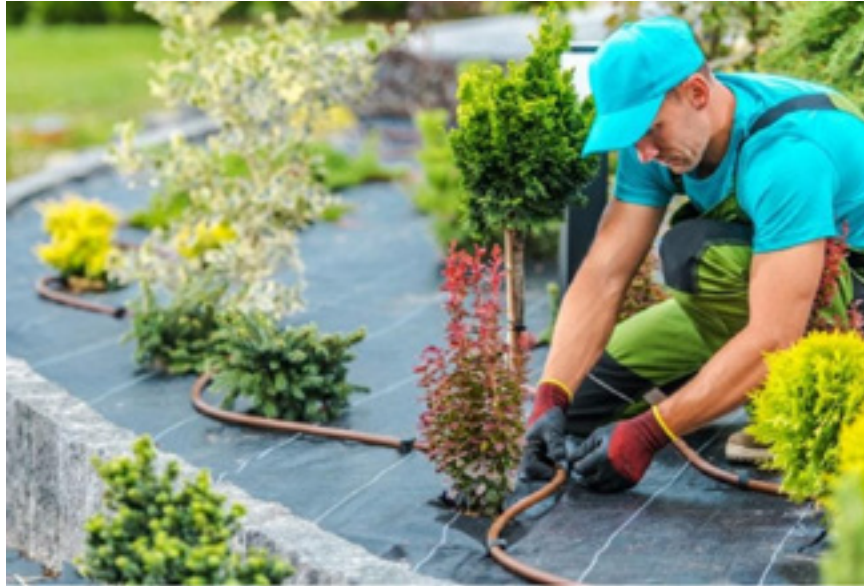
Drip lines installed in planting bed prior to mulching to hide lines.
