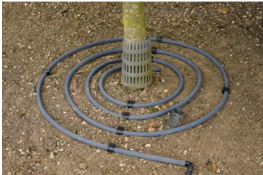
Individual tree drip line for deep root watering. These lines are concealed with 3-inch layer mulch ring.
