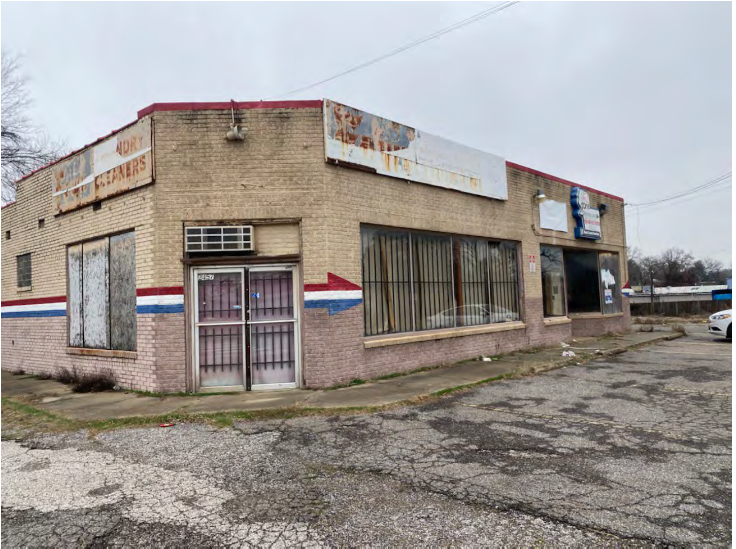
View of structure from corner
