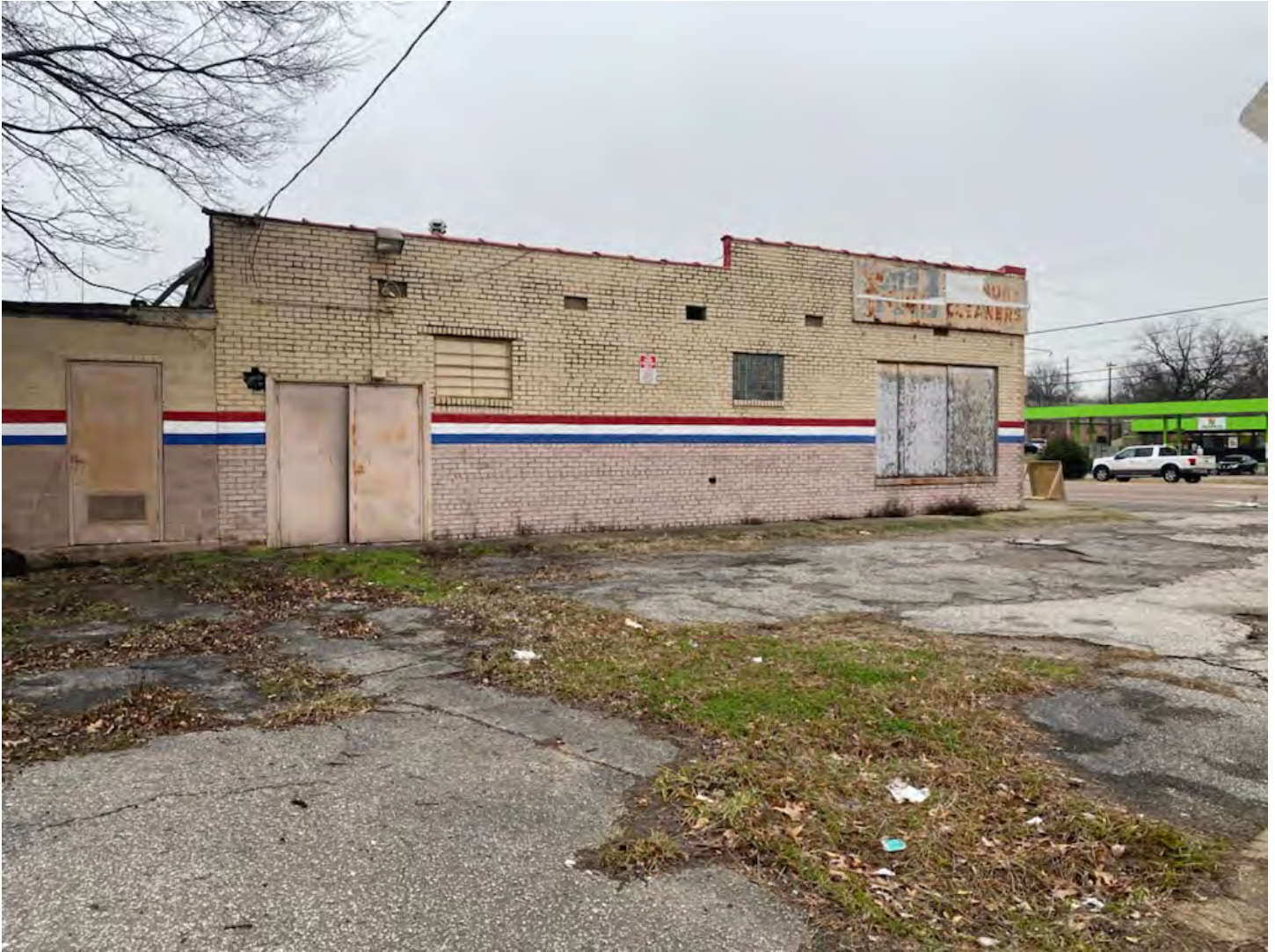
View of structure from Alcy
