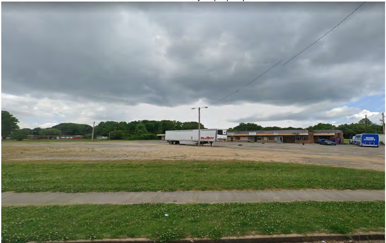
Abandoned shopping center on the other side of Horn Lake from subject property zoned CMU-1 4777 Horn Lake Rd
