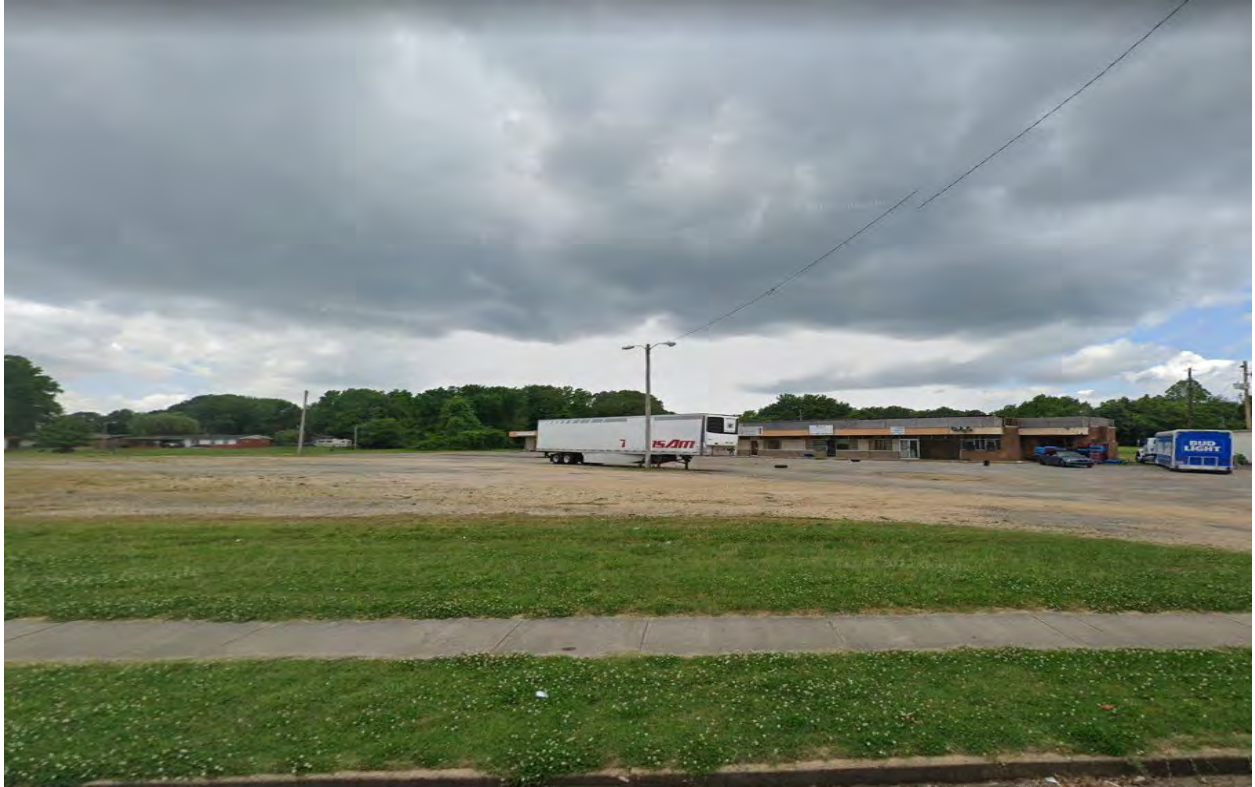
Abandoned shopping center on the other side of Horn Lake from subject property zoned CMU-1 4777 Horn Lake Rd
