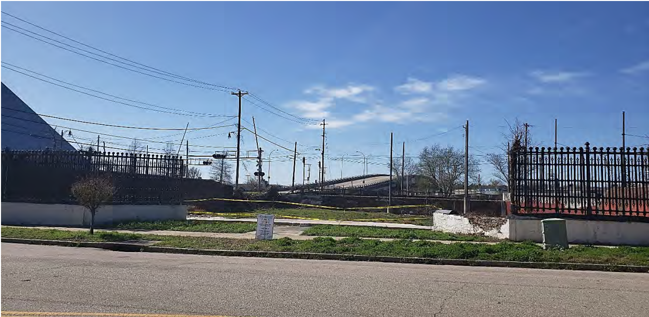
View of subject property from North Front Street looking southwest
