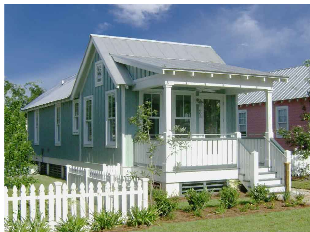
EXAMPLE OF MERIGOLD COTTAGE
