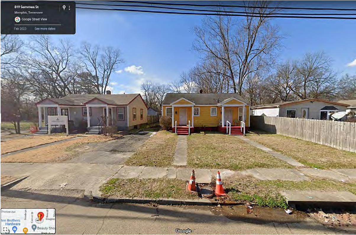
View from subject property looking west
