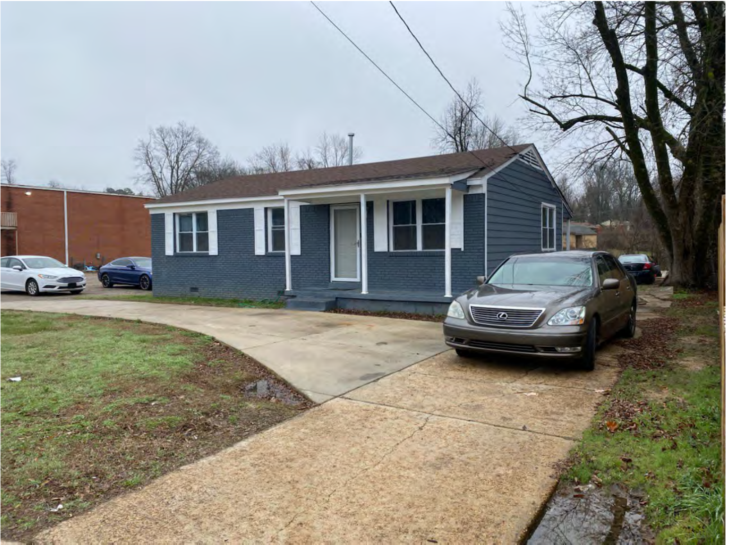
View of existing structure from Frayser
