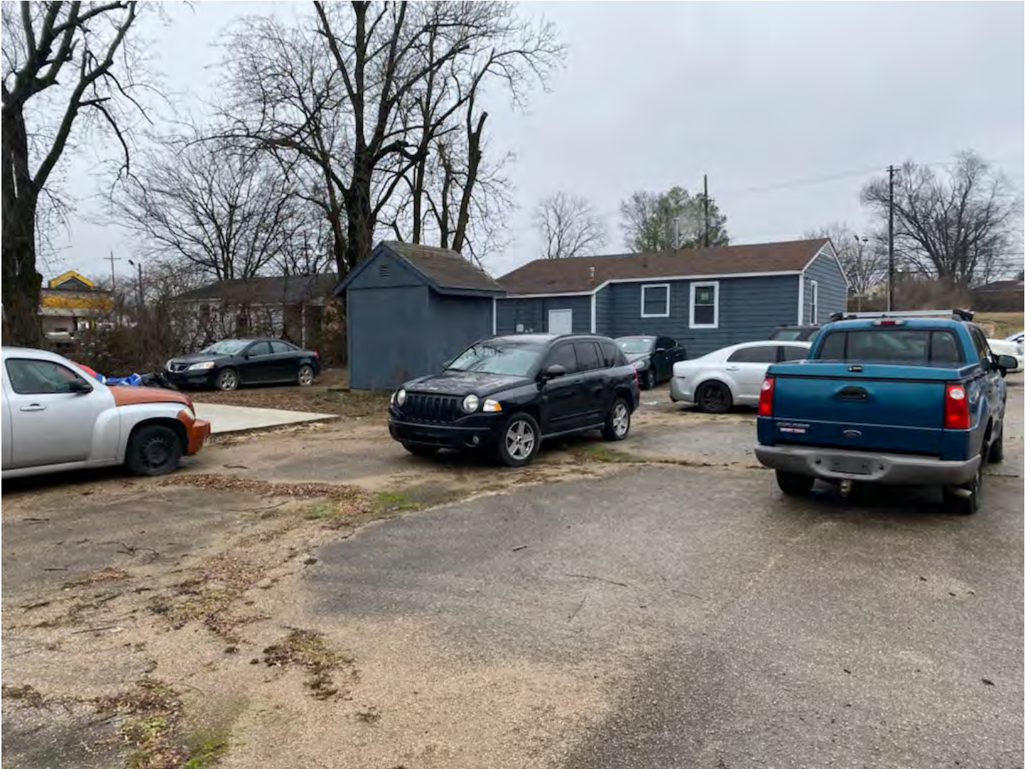
Rear of existing structure
