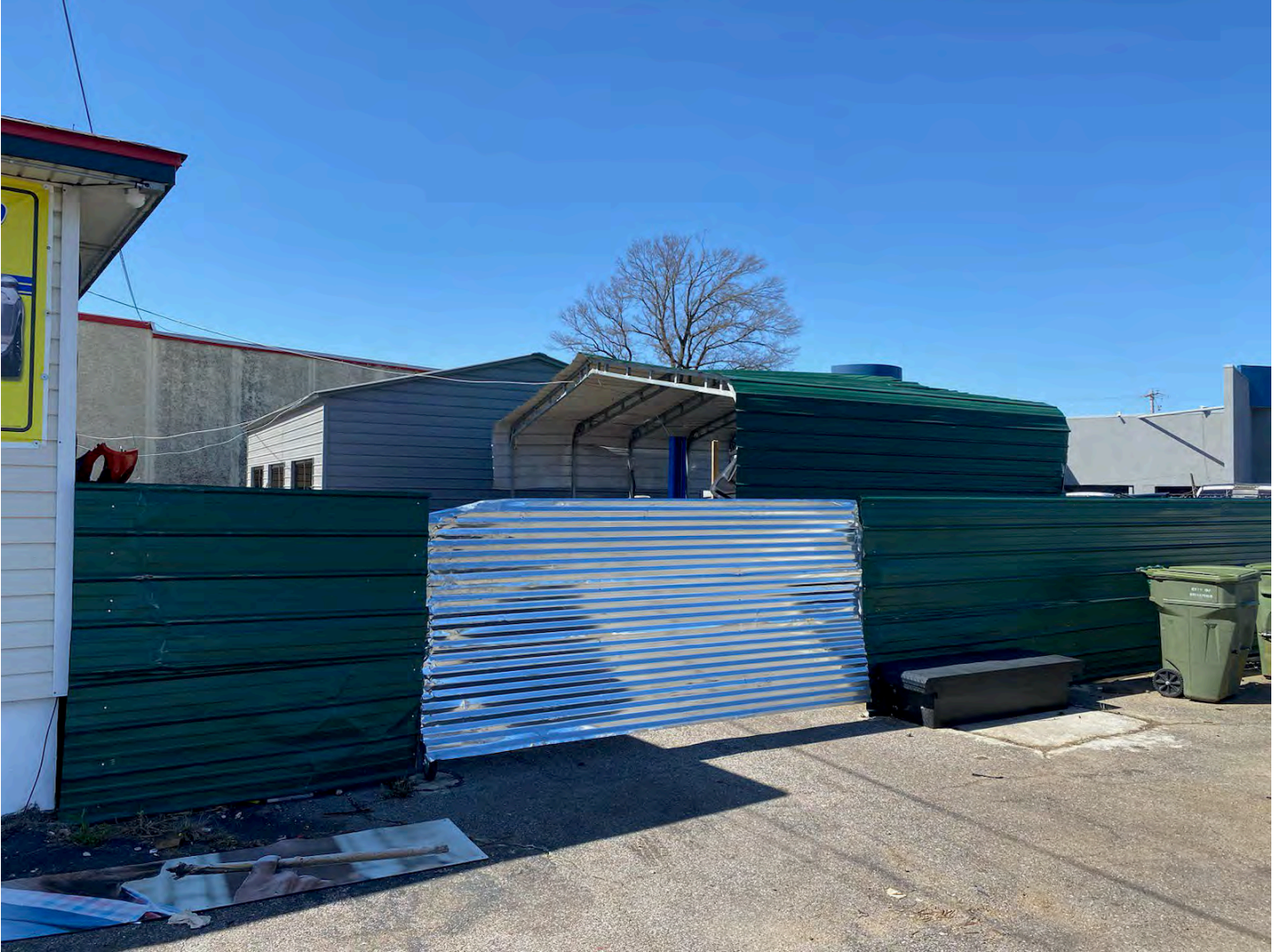
Existing metal fence and two accessory structures (carport and garage)
