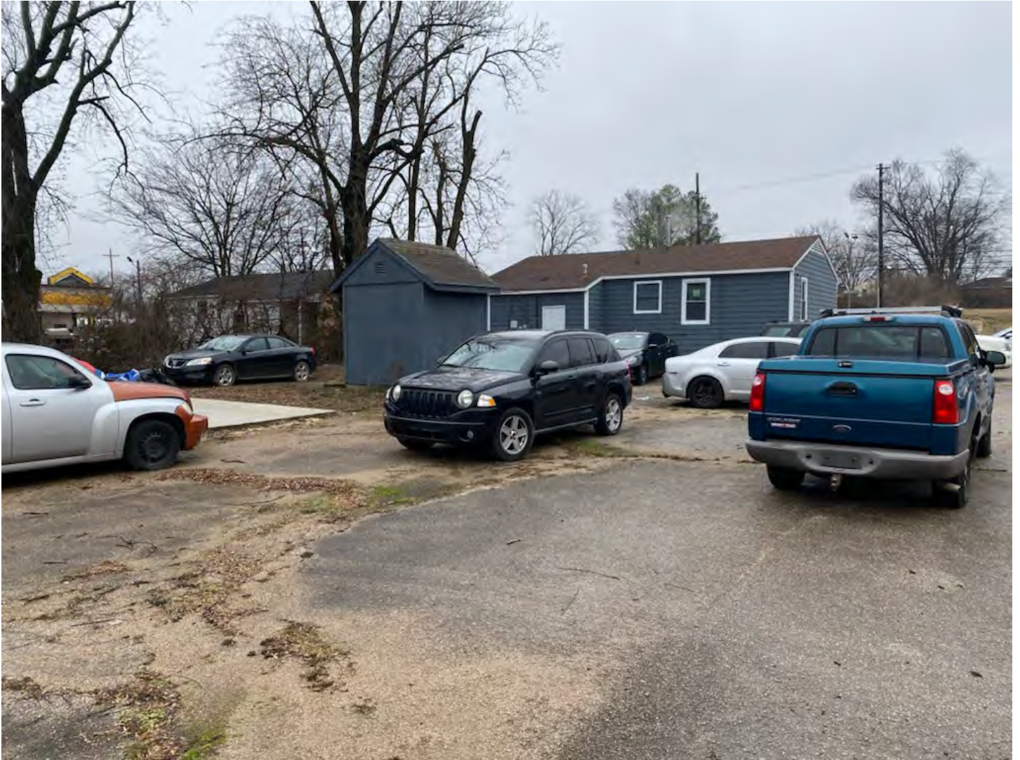
Rear of existing structure
