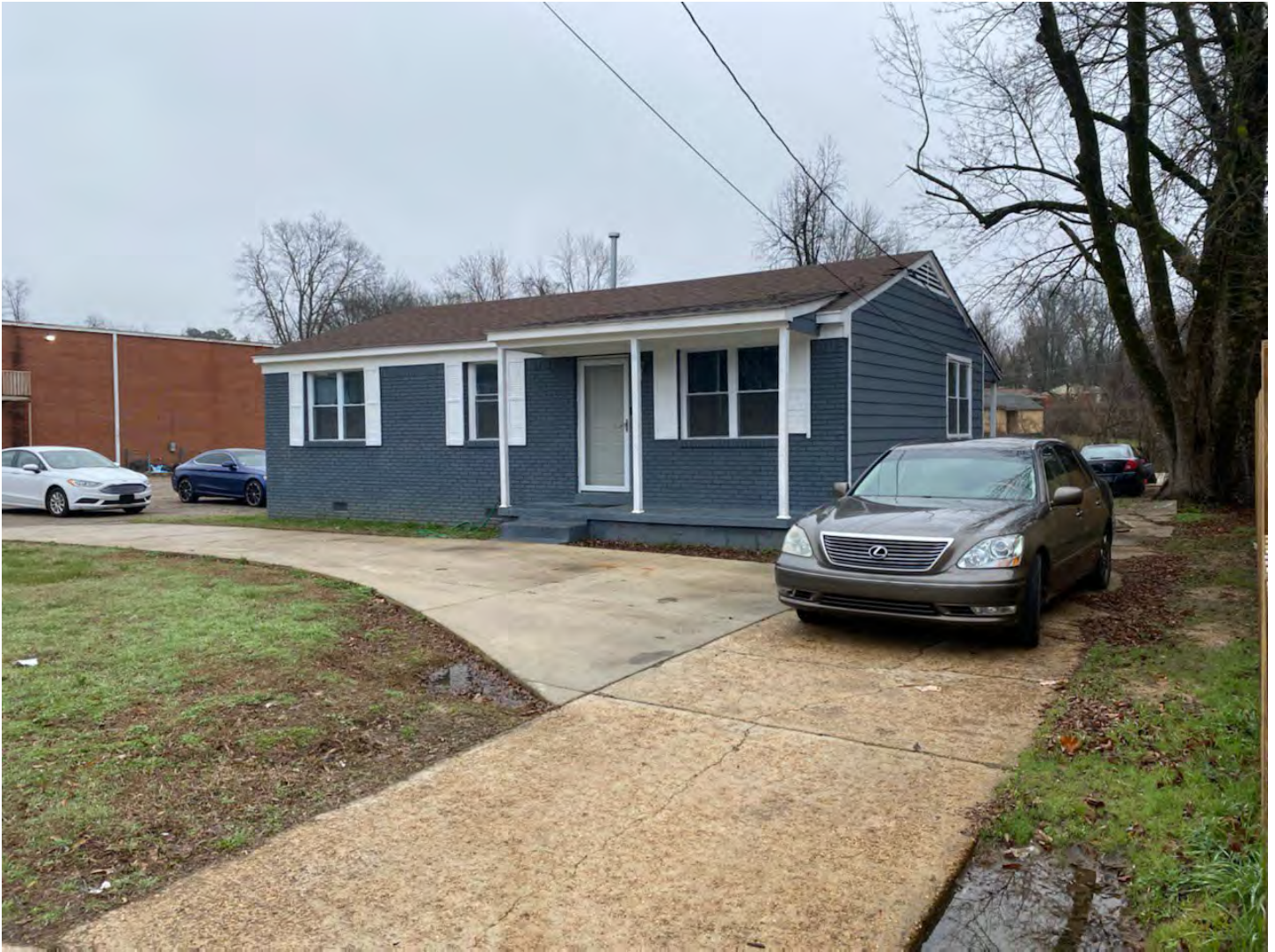
View of existing structure from Frayser
