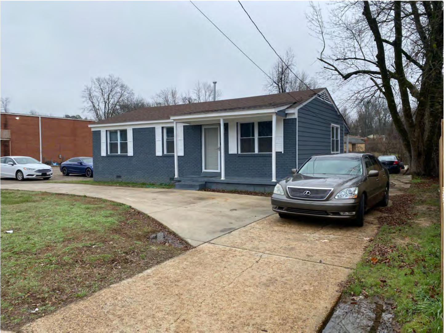
View of existing structure from Frayser
