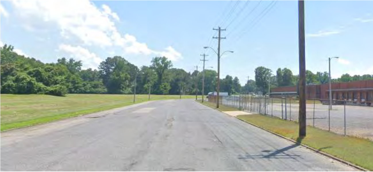
View of access point/ intersection of Durham Avenue and Steele Street looking west
