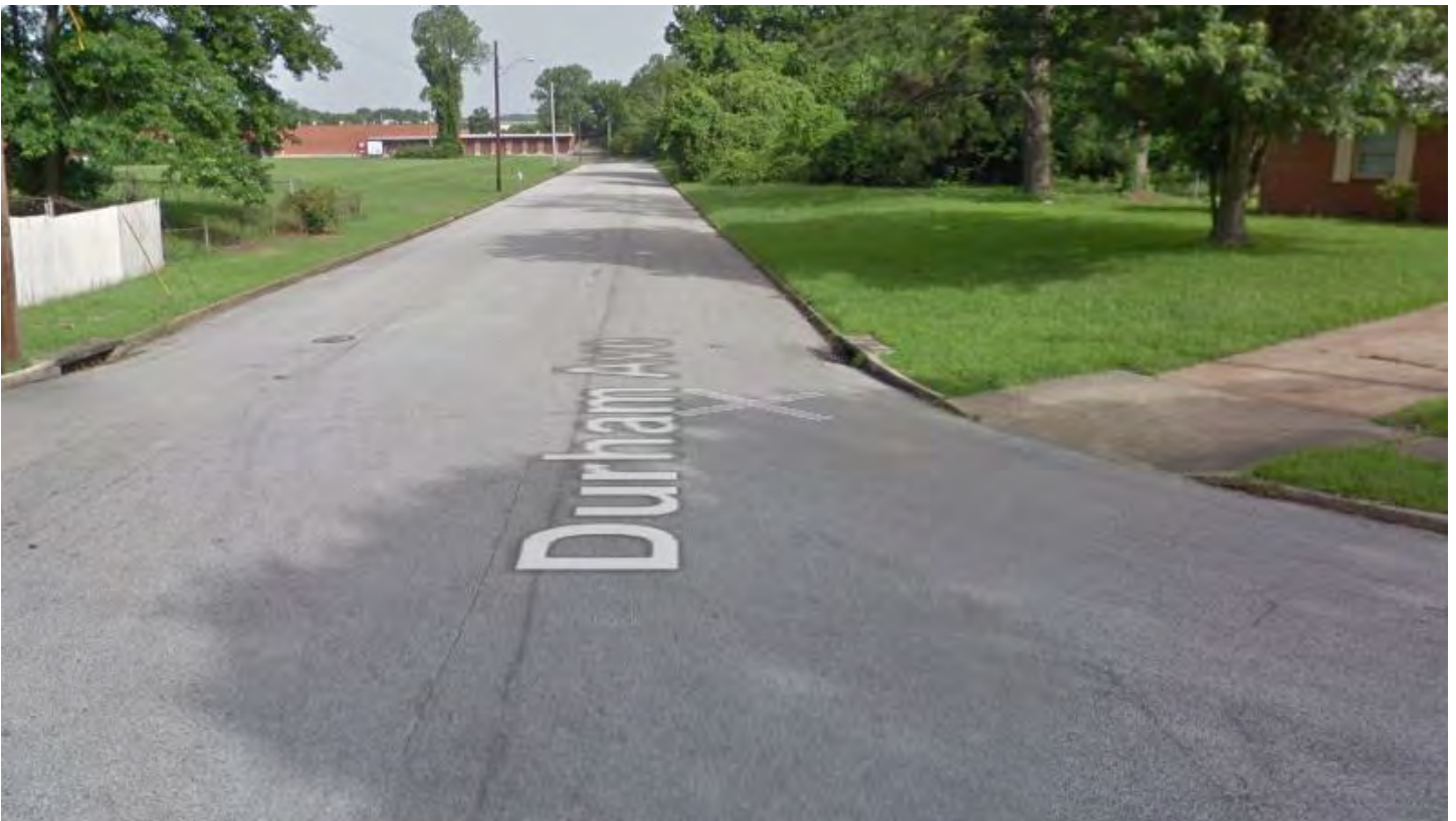
View of access point Durham Avenue from Argonne Street looking North
