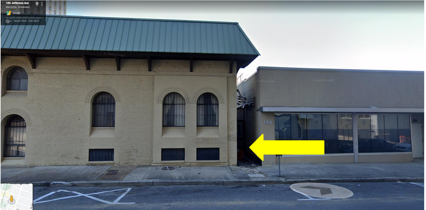
View of access point (yellow arrow) to unnamed public alley from Jefferson Avenue looking north
