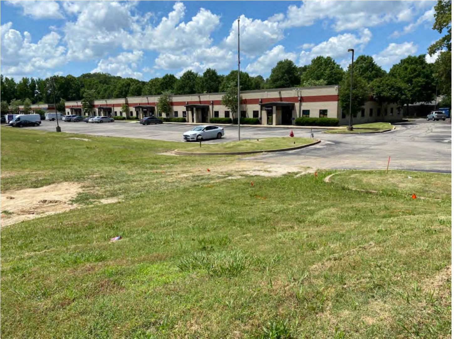
View of adjacent office building
