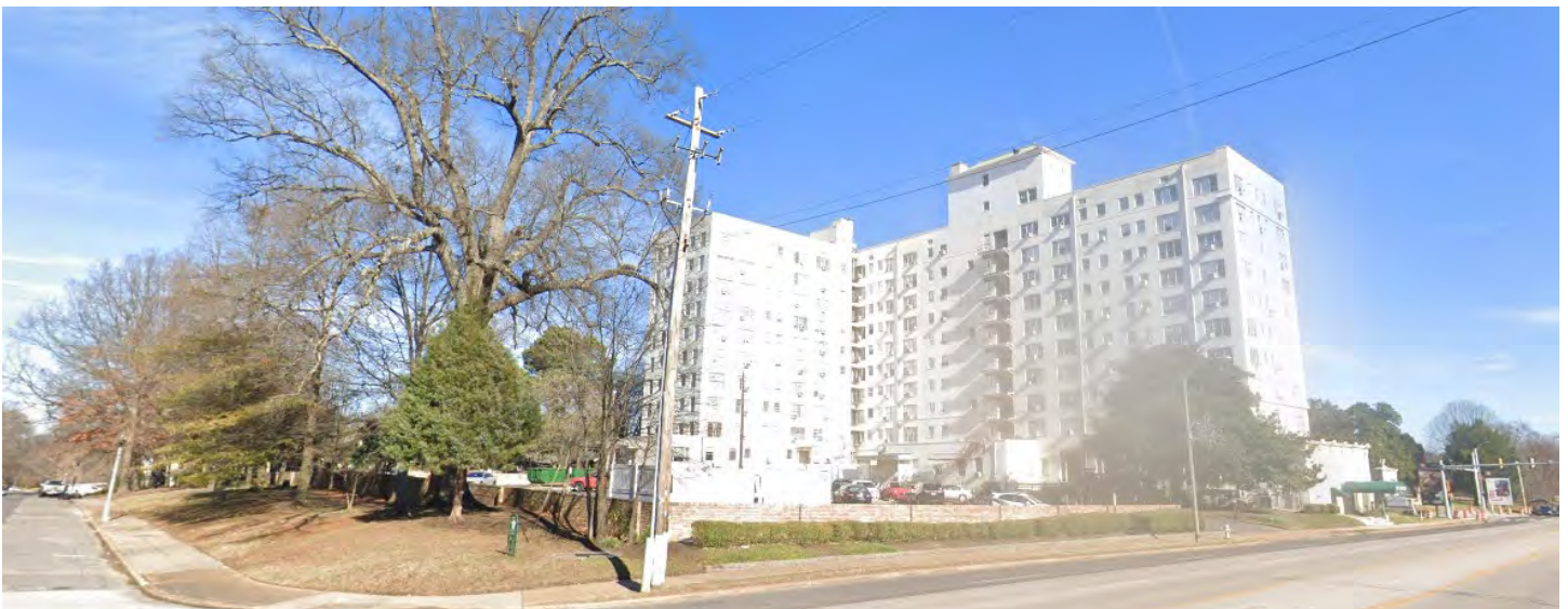
View of the subject property from Poplar Avenue looking northeast
