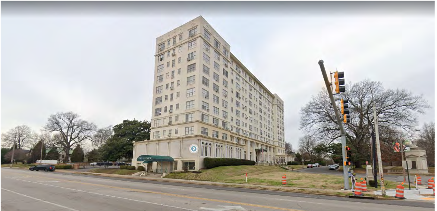
View of the subject property from Poplar Avenue looking north
