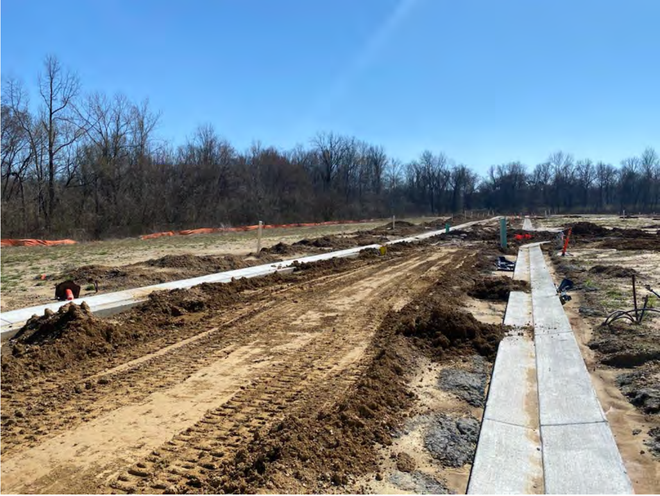
Road construction at Phase 3
