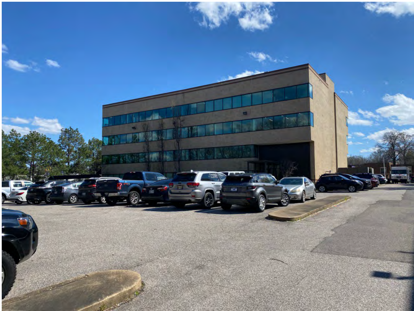
The rear of the adjacent office building
