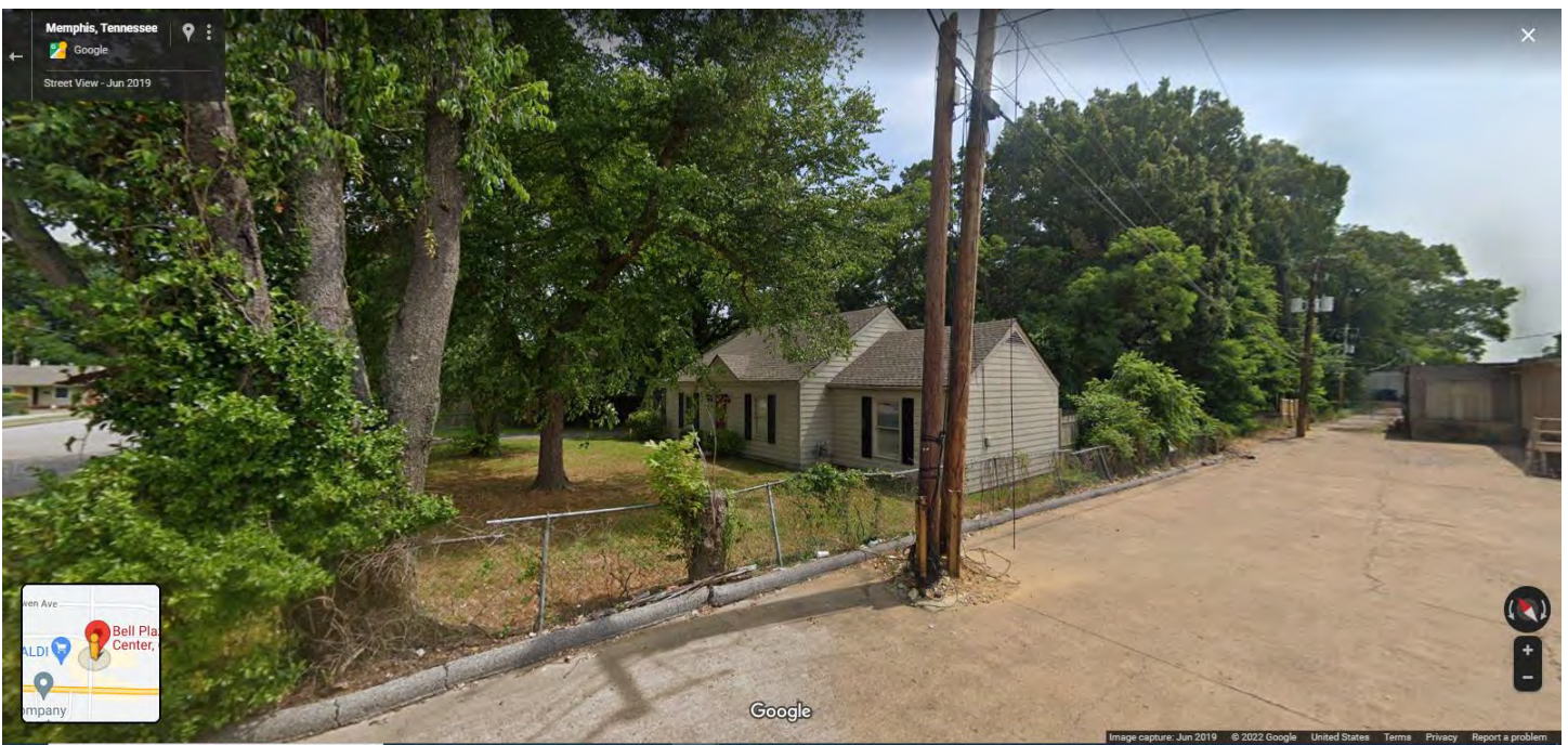
View of subject property from a commercial parking lot facing northeast.
