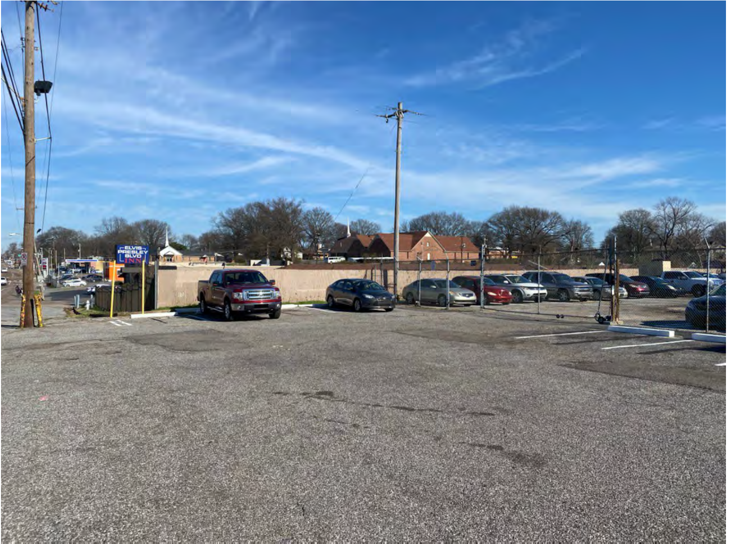
An alternative view of the rear parking area.
