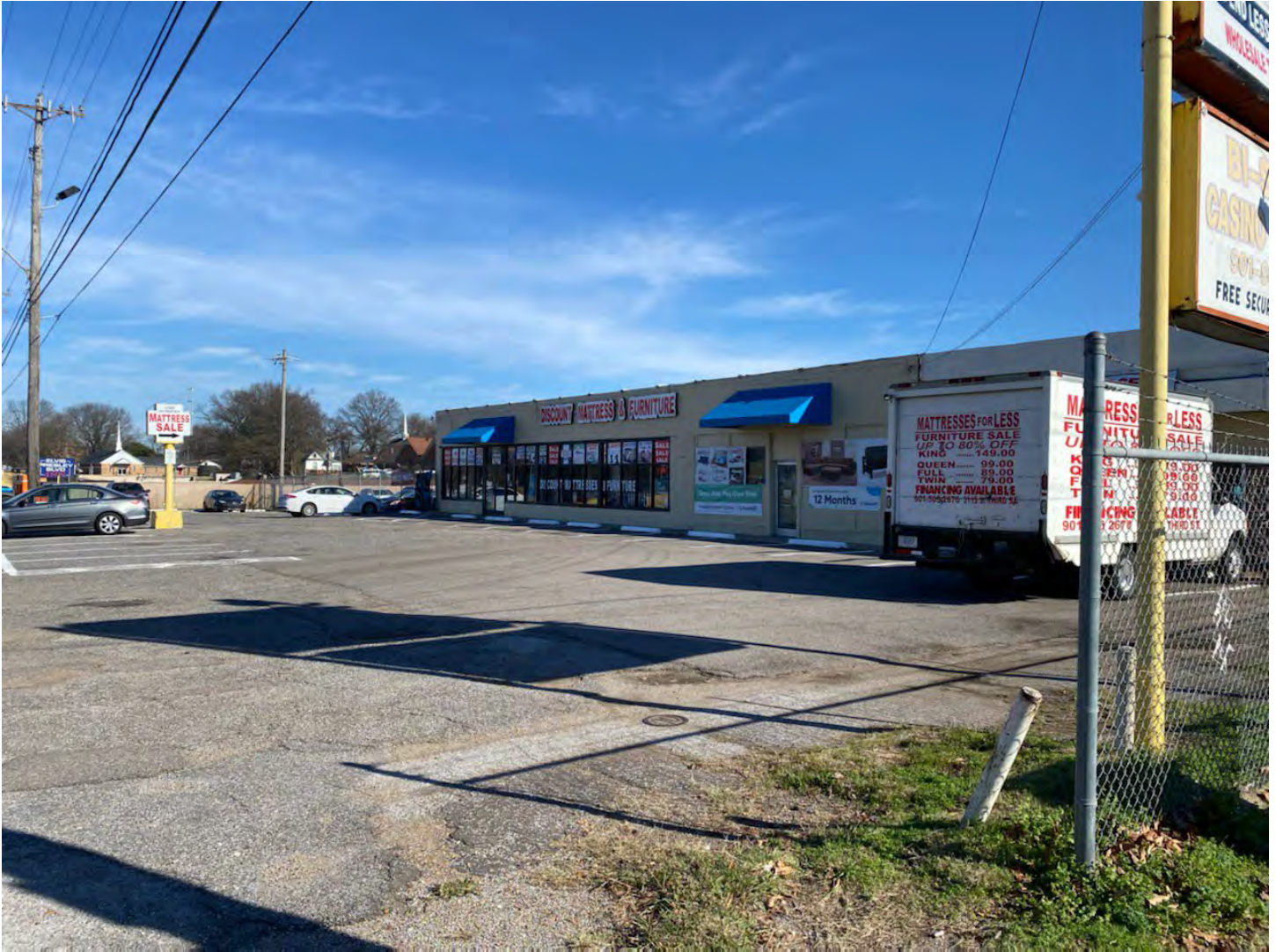
A view of the shopping strip, including the furniture store (left) and a vacant storefront (right). Note the truck, two detached signs, and chain link fencing.
