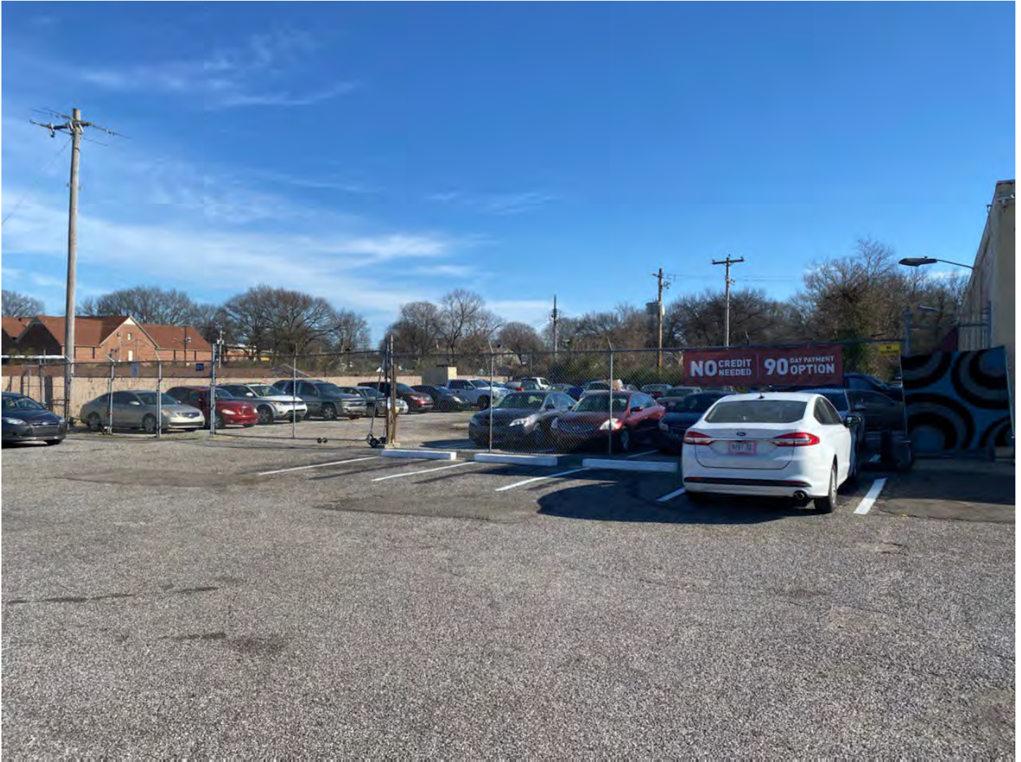
A view of the rear parking area. Note the chain link fencing and gate, as well as signage on fence.
