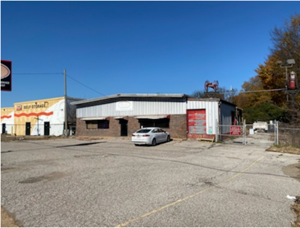
The principal structure
