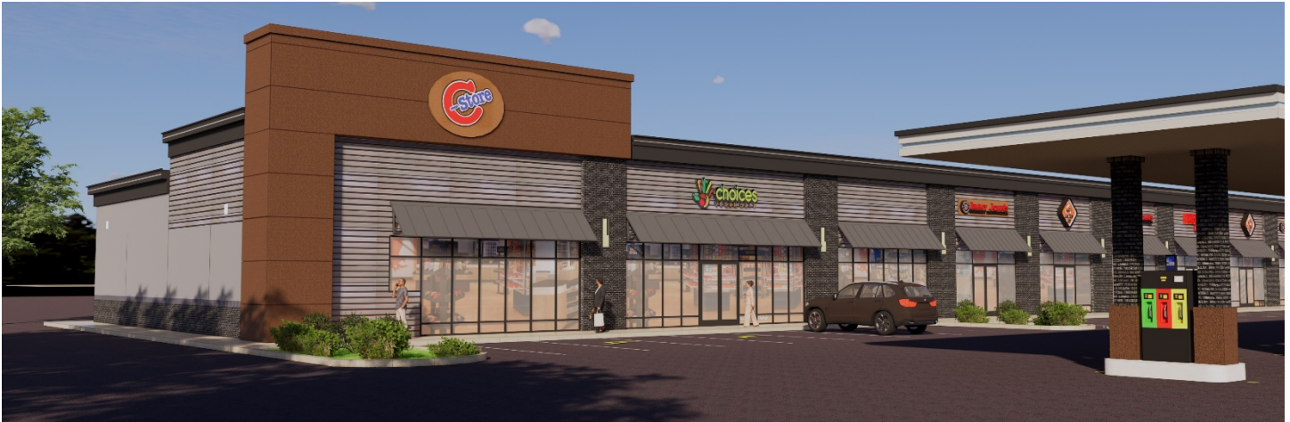
View of C store from street
