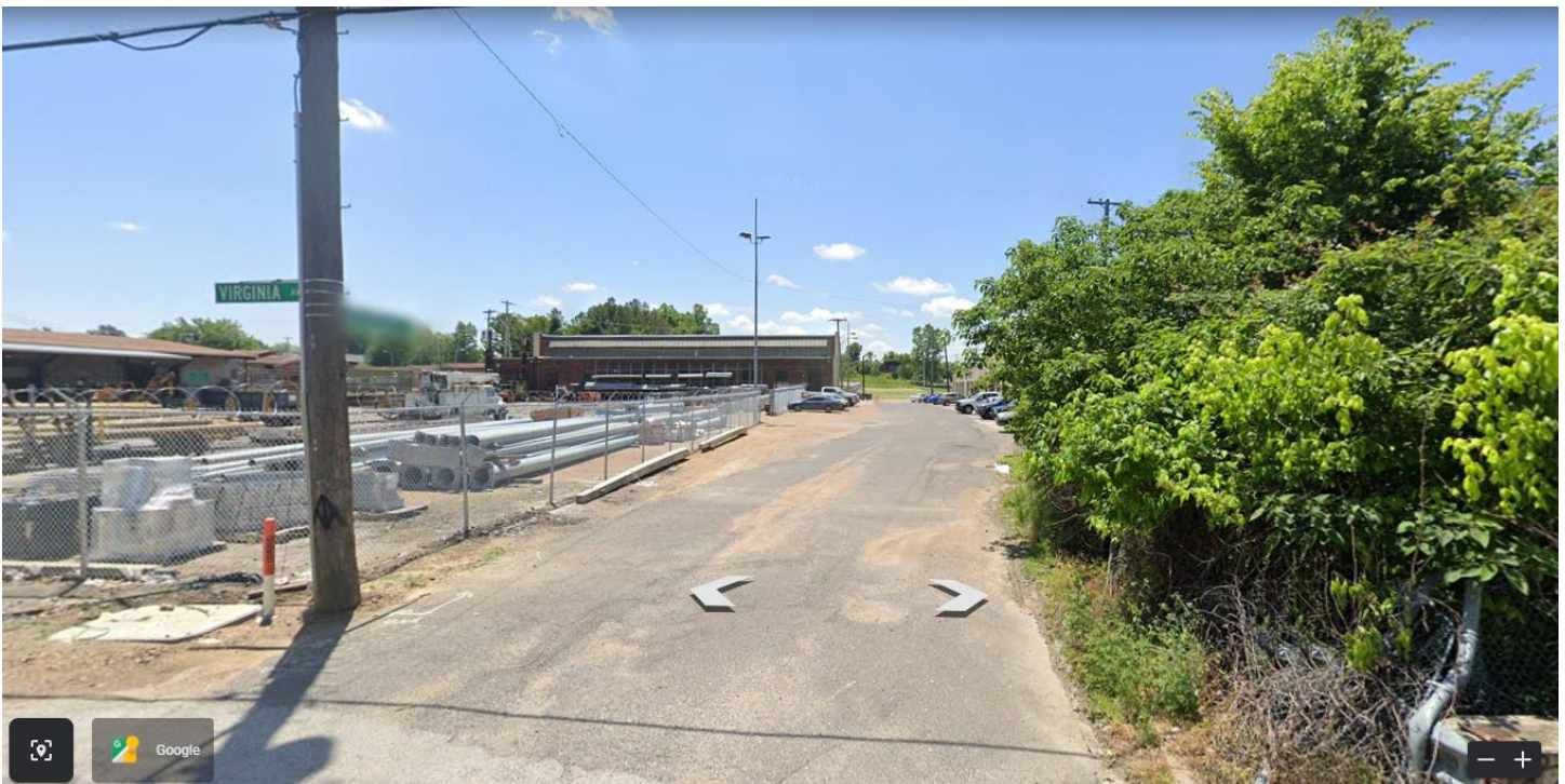
View of access point to the subject right-of-way from the East Virginia Avenue facing south
