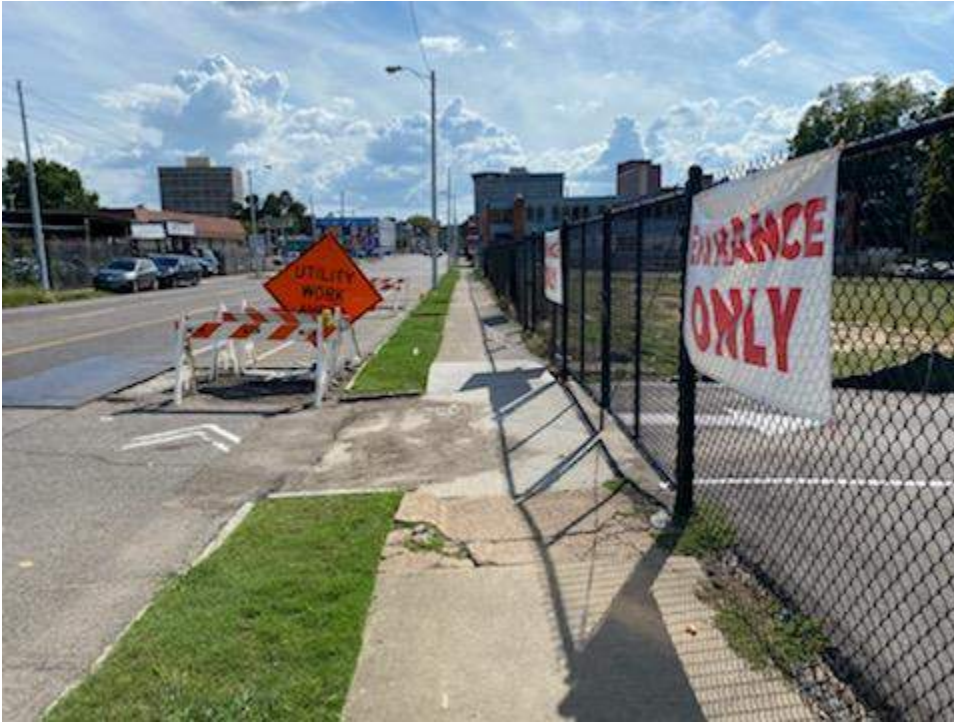
A view south down Cleveland. The subject right-of-way lines up with the curb cut.
