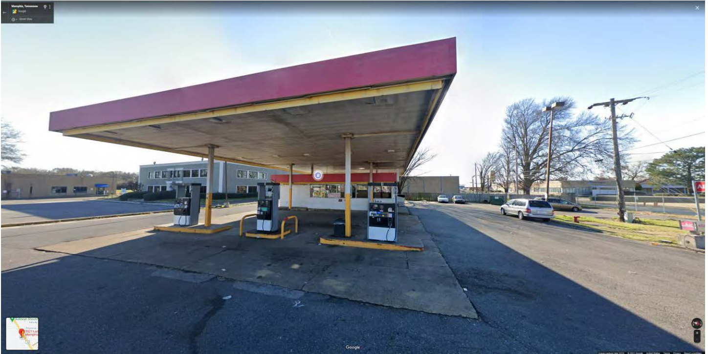
View of the current pump configuration and principle structure facing west
