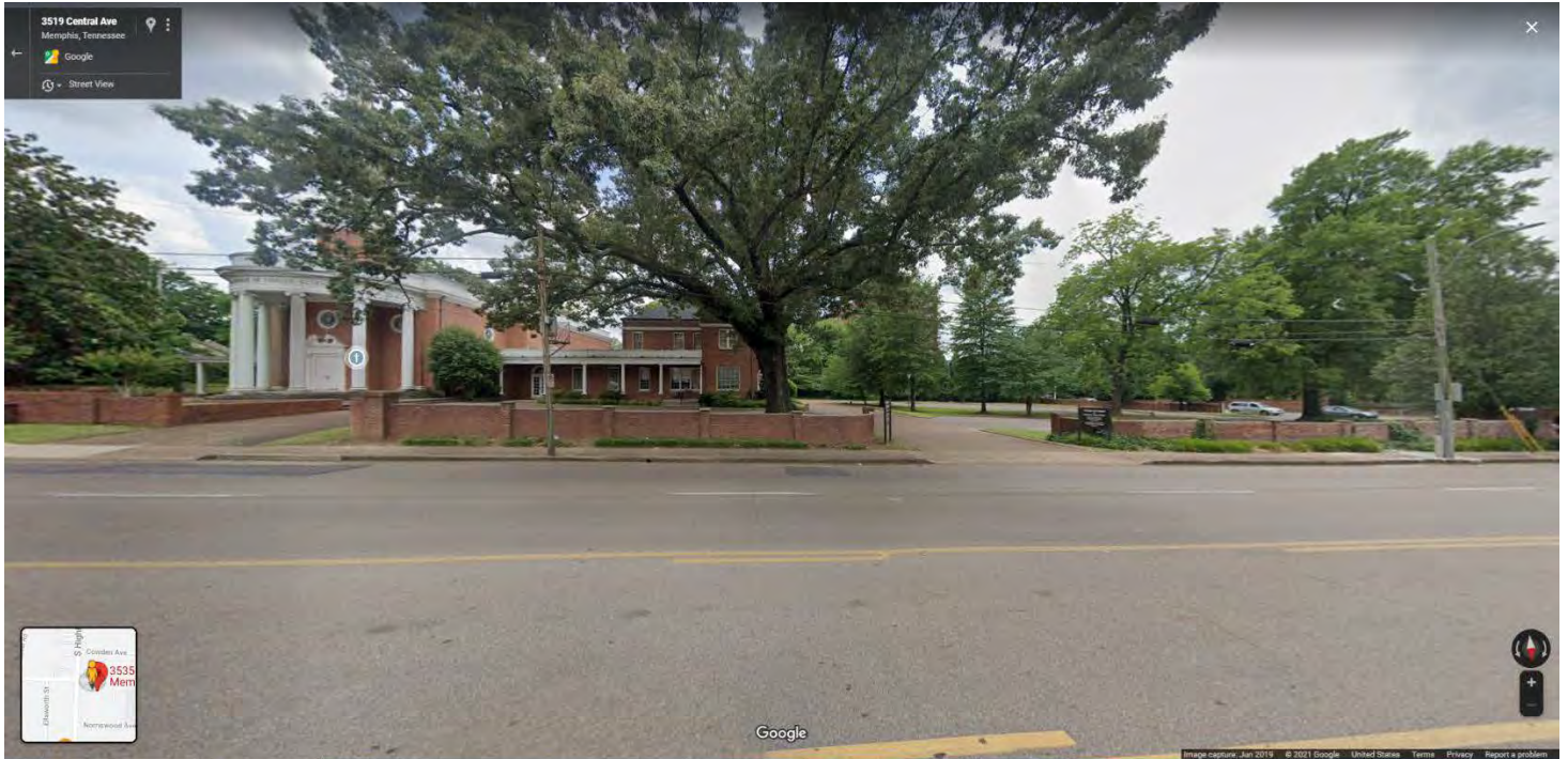
View of subject property from Central Avenue looking south
