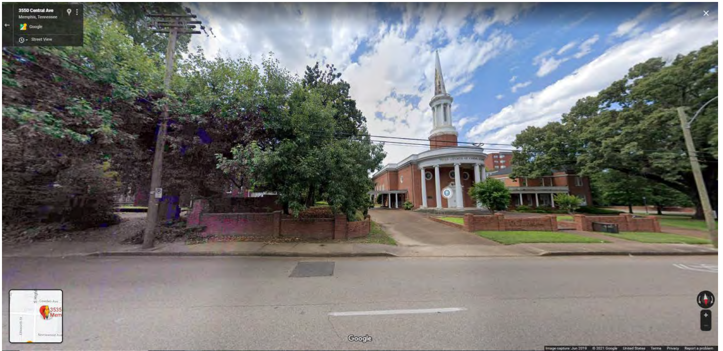
View of subject property from Central Avenue looking south
