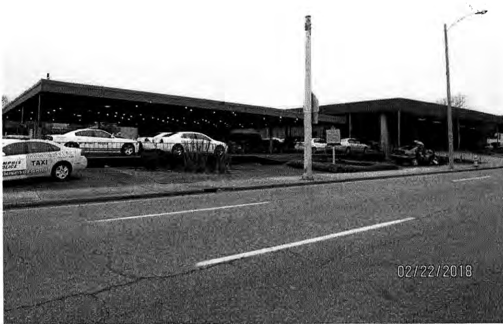
Front view – looking southwest from Union Avenue
