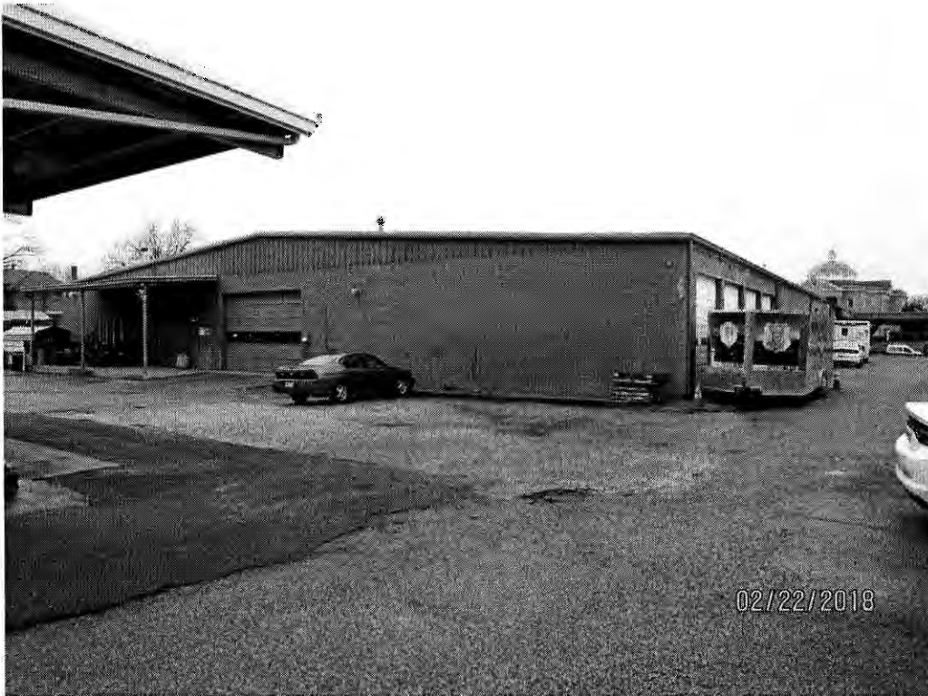
Rear view – looking north
