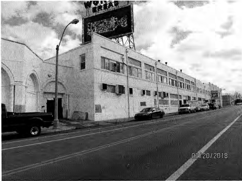
0 Monroe Avenue Northeast corner of Monroe Avenue and Danny Thomas Boulevard Tax Parcel ID: 7-1-4C
