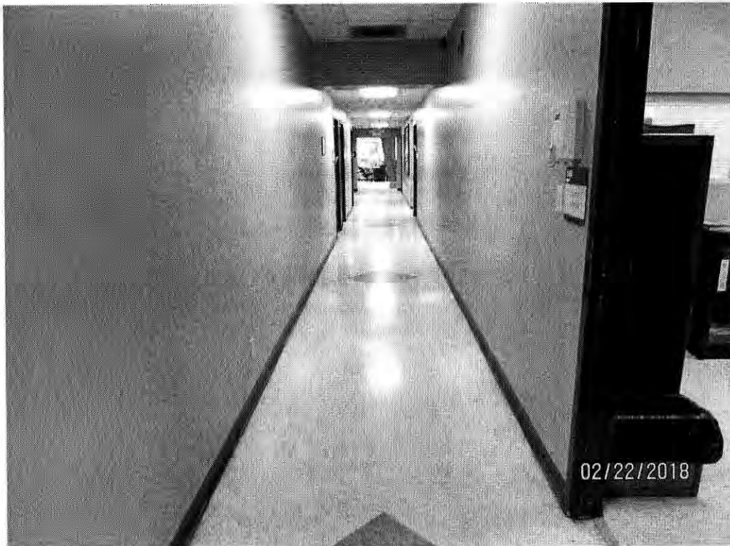
Typical view of hallway
