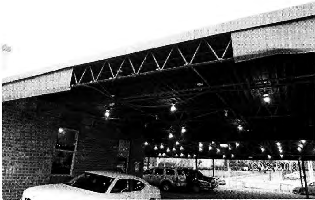
Deferred maintenance – missing metal
