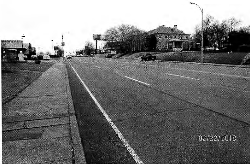
Typical Street Scene – Looking west along Union Avenue – subject property on left
