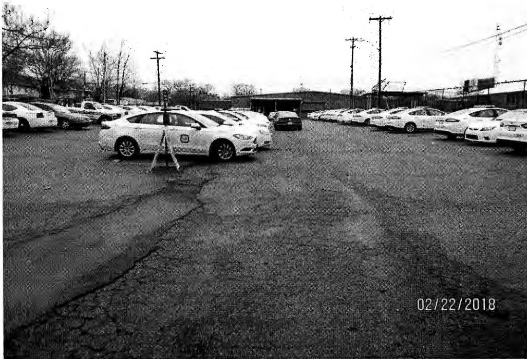
Typical interior view – looking north from south property line
