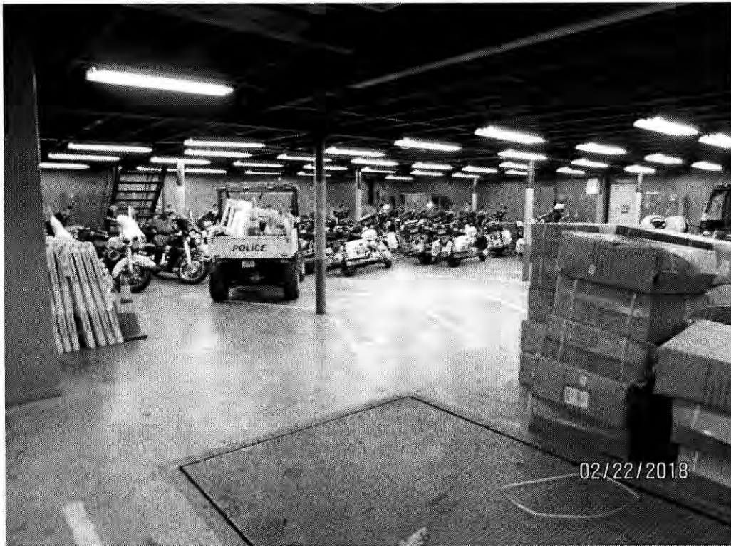
Spare motor bay interior
