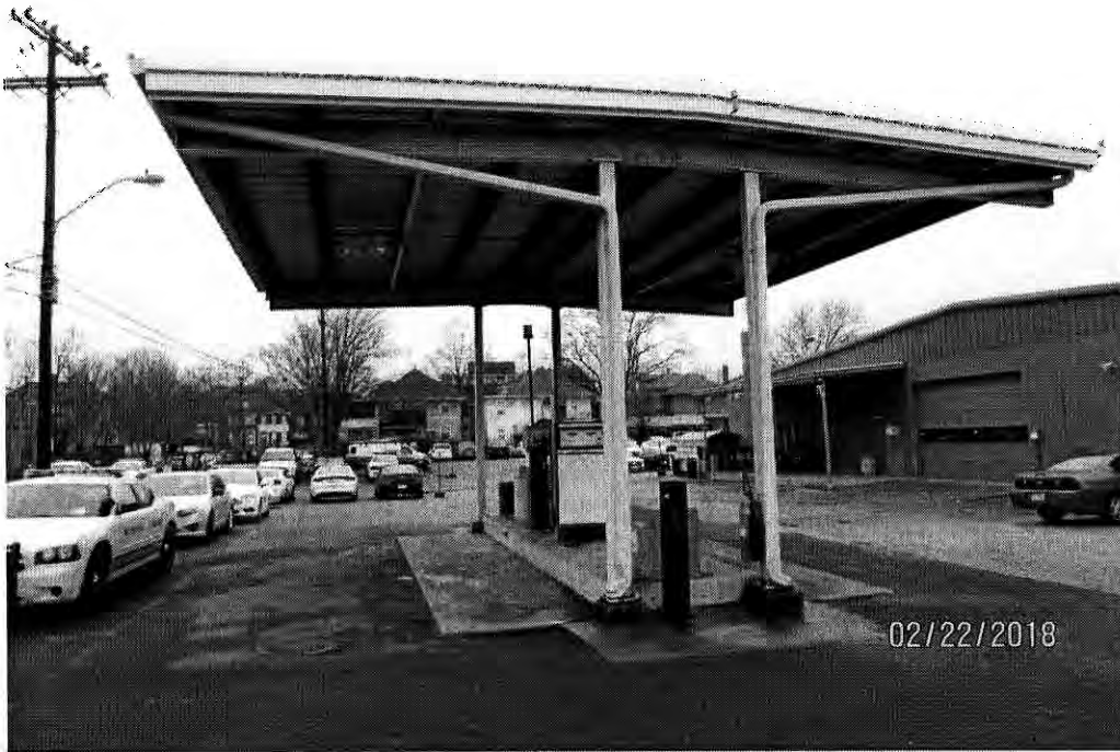
Gas pump and canopy
