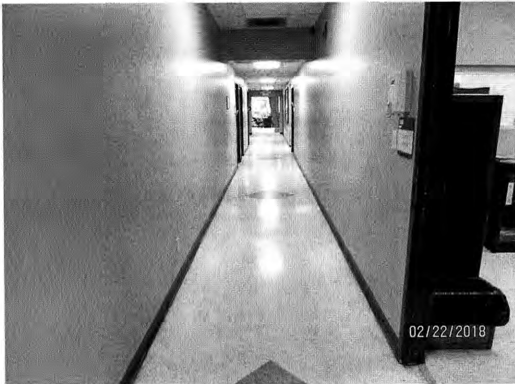
Typical view of hallway
