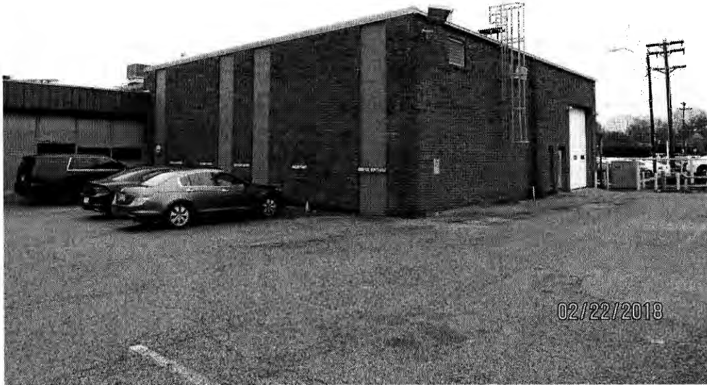
Spare motor bay on west side – looking southeast
