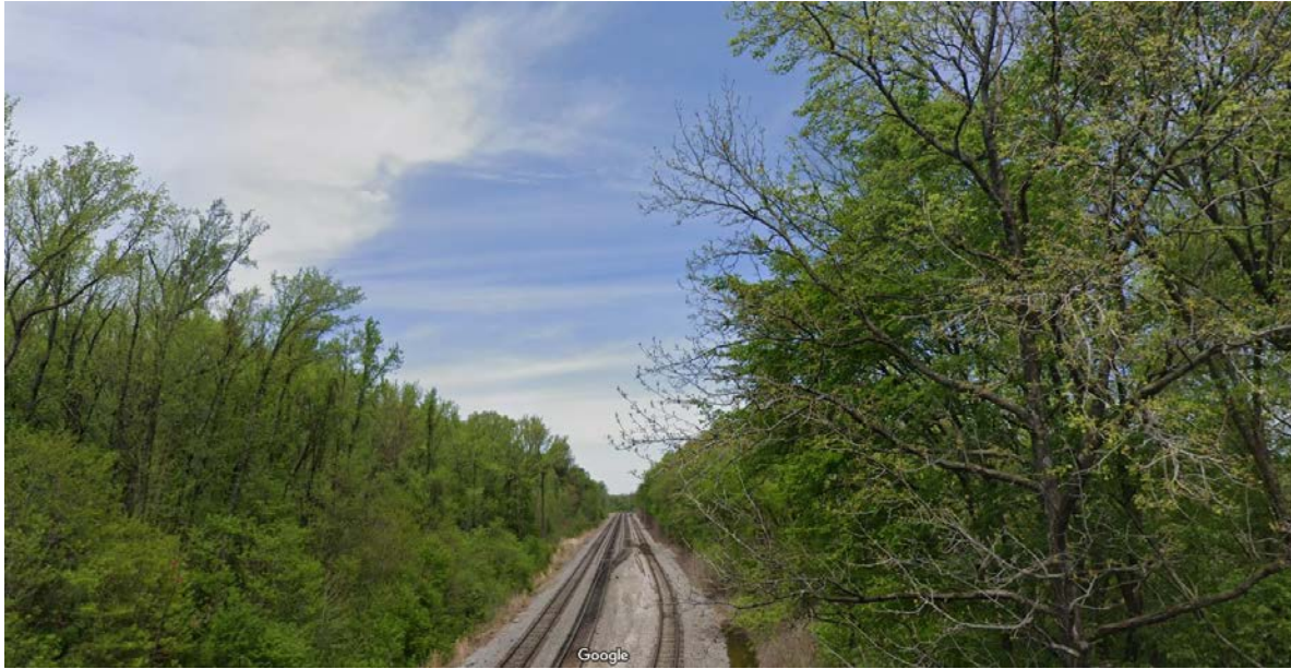
Much of the proposed route will follow these Canadian National (formerly Illinois Central) tracks through Southwest Memphis.
