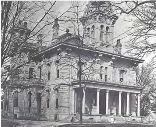
Henry A. Montgomery home 1200 Poplar Avenue
