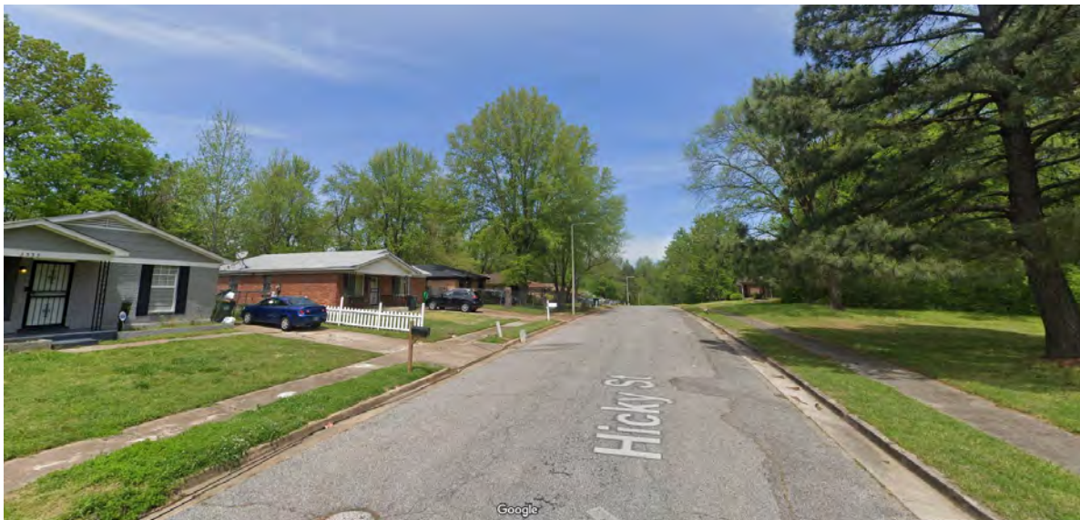
View looking north along Hicky Street in the Hicky subdivision; the proposed pipeline would be located within railroad right-of-way behind the homes on the left.
