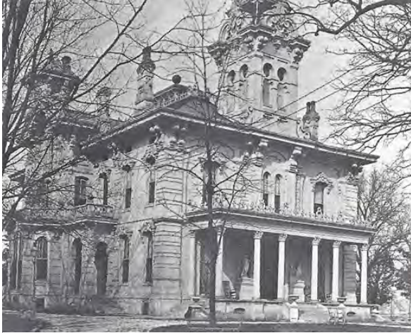
Henry A. Montgomery home 1200 Poplar Avenue
