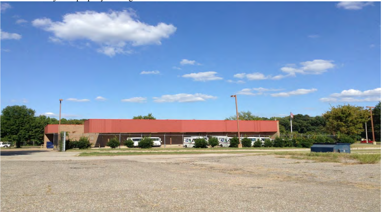
Front view of adjacent property to the east of subject property
