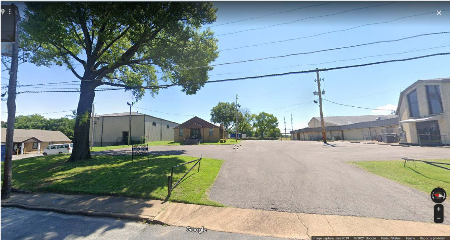
View of west side (front) of subject property looking east
