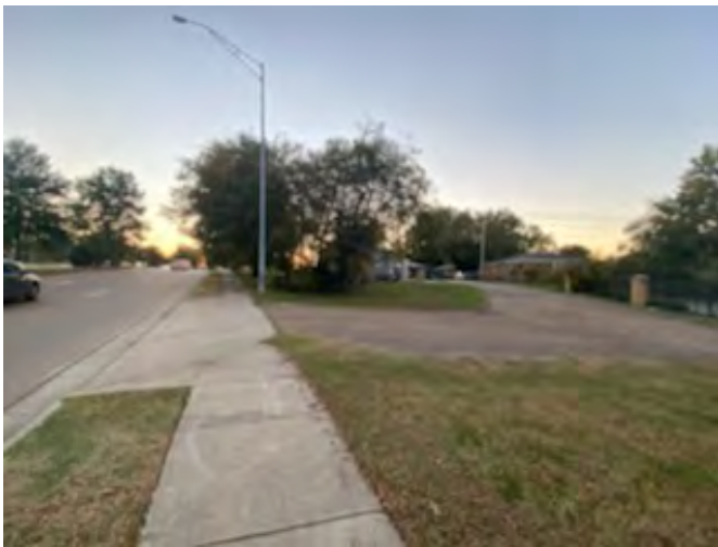
View of existing ingress/egress between Sam Cooper and subject right-of-way.
