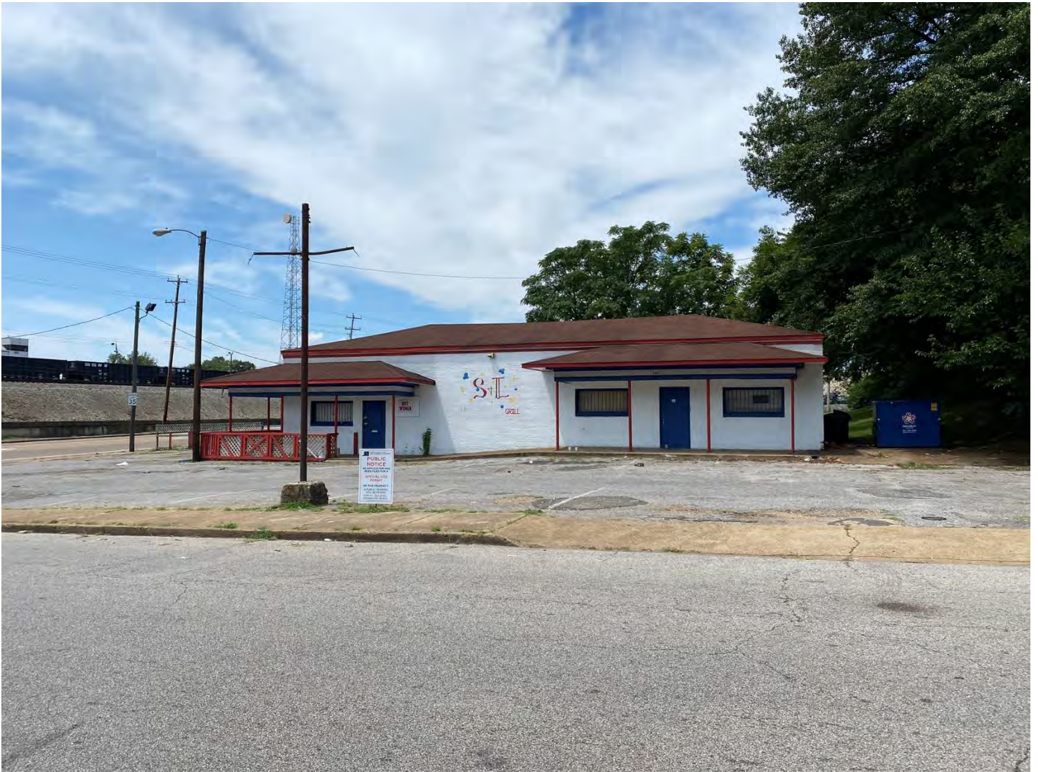
View of subject structure – a vacant restaurant – from Boston
