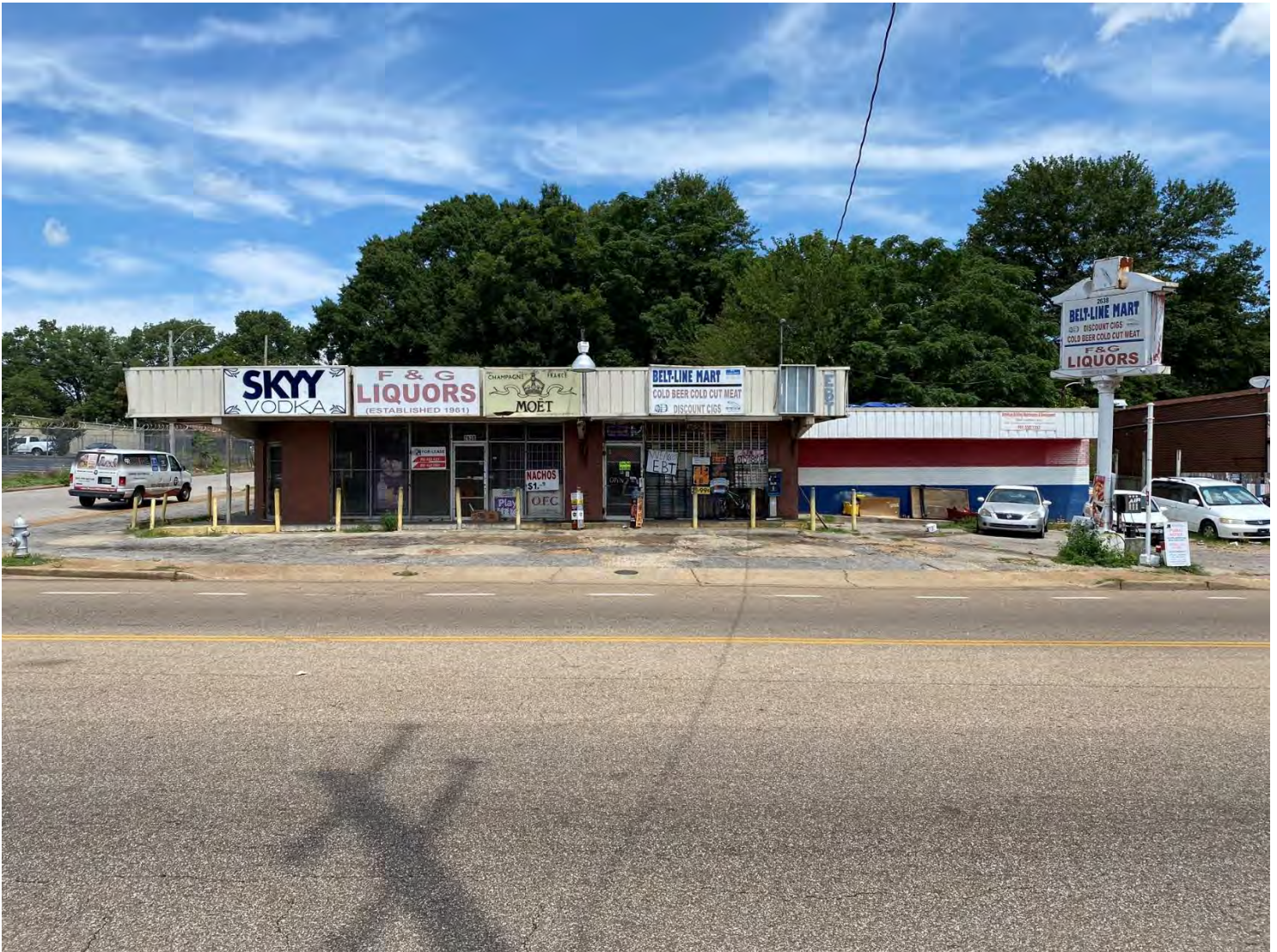
A view of subject structures from Southern
