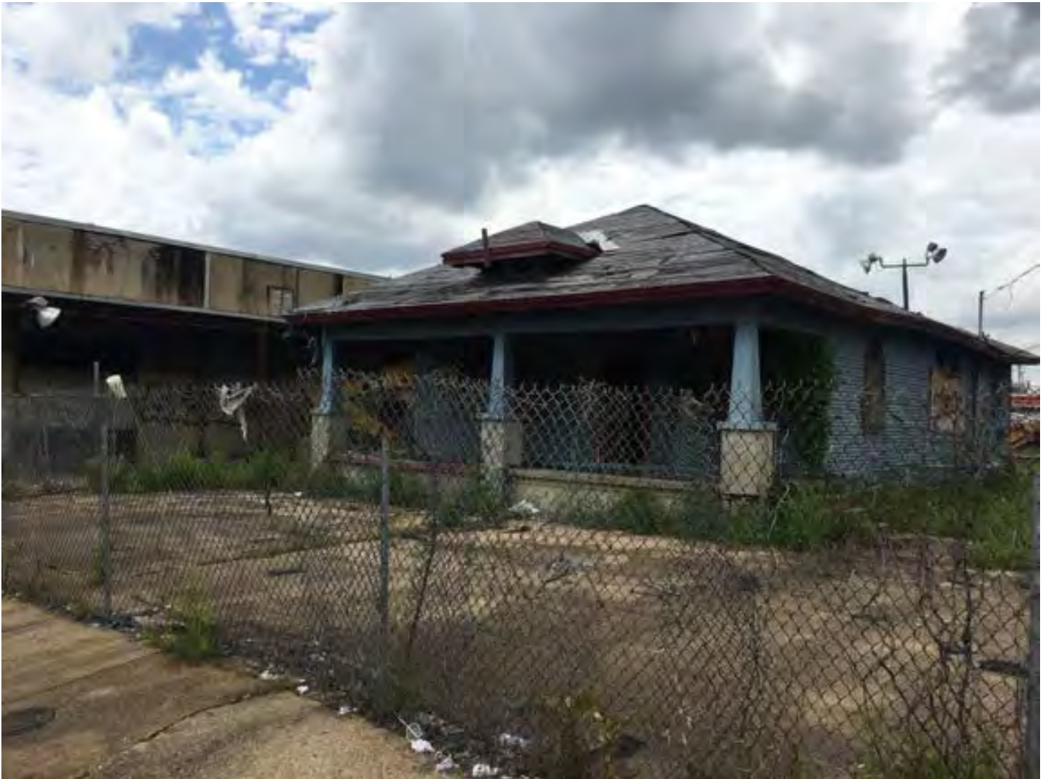
View of a subject structure on west side of Malcomb
