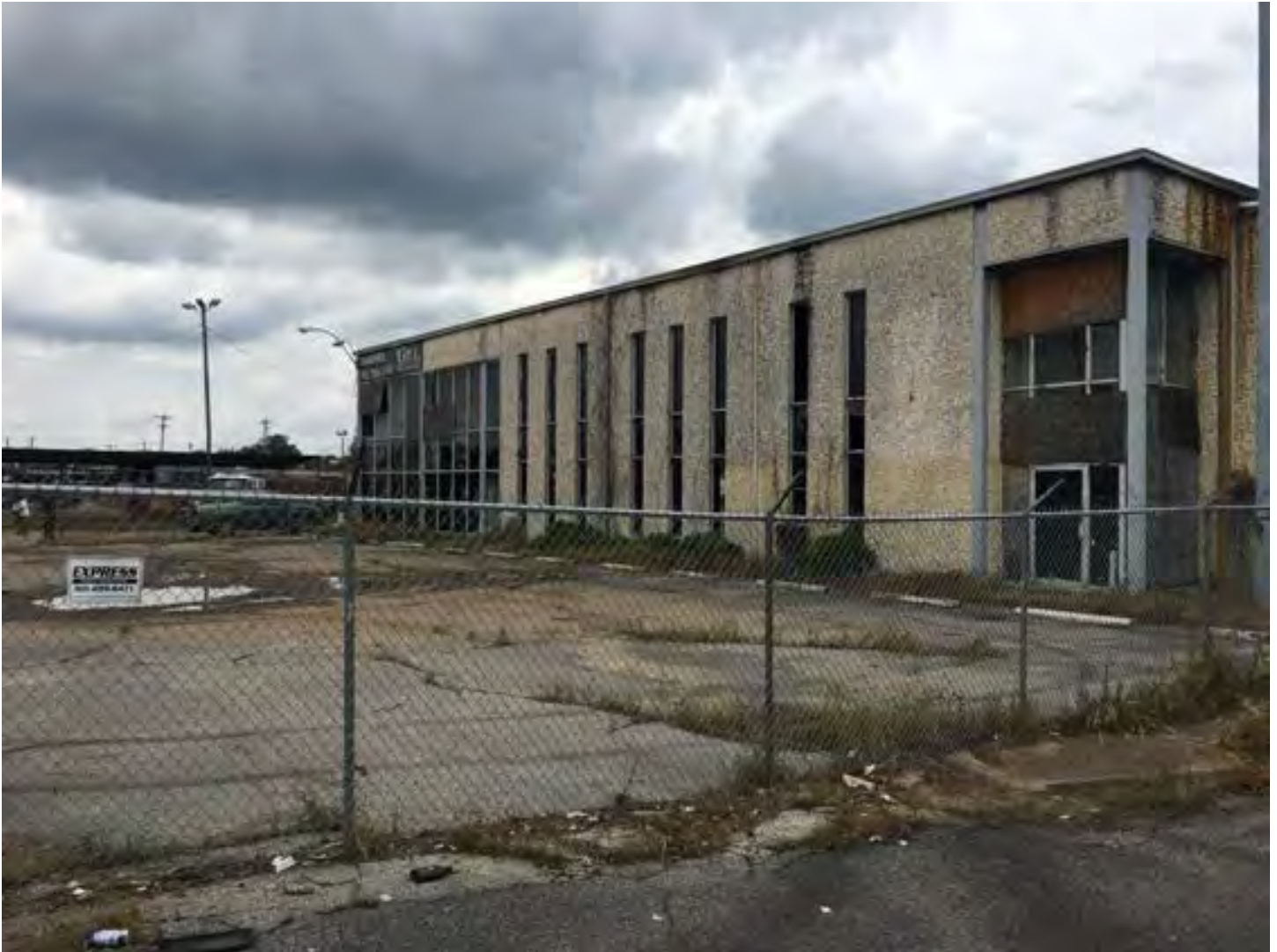
View of a subject structure from Malcomb
