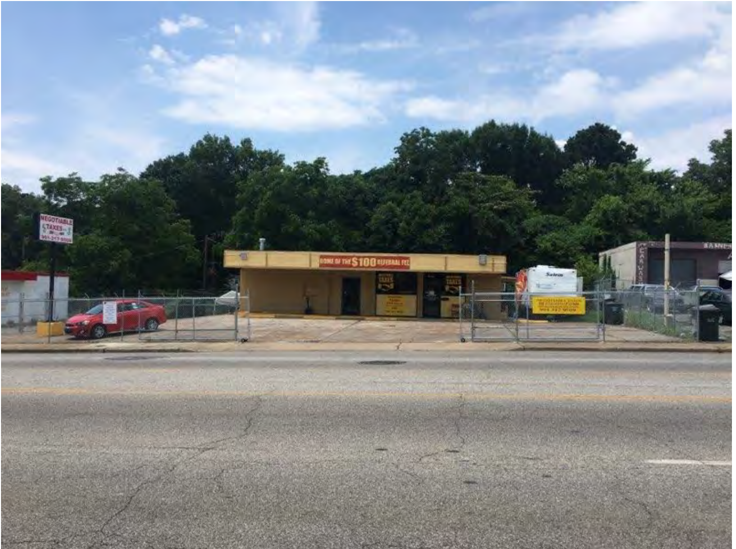
View of subject lot
