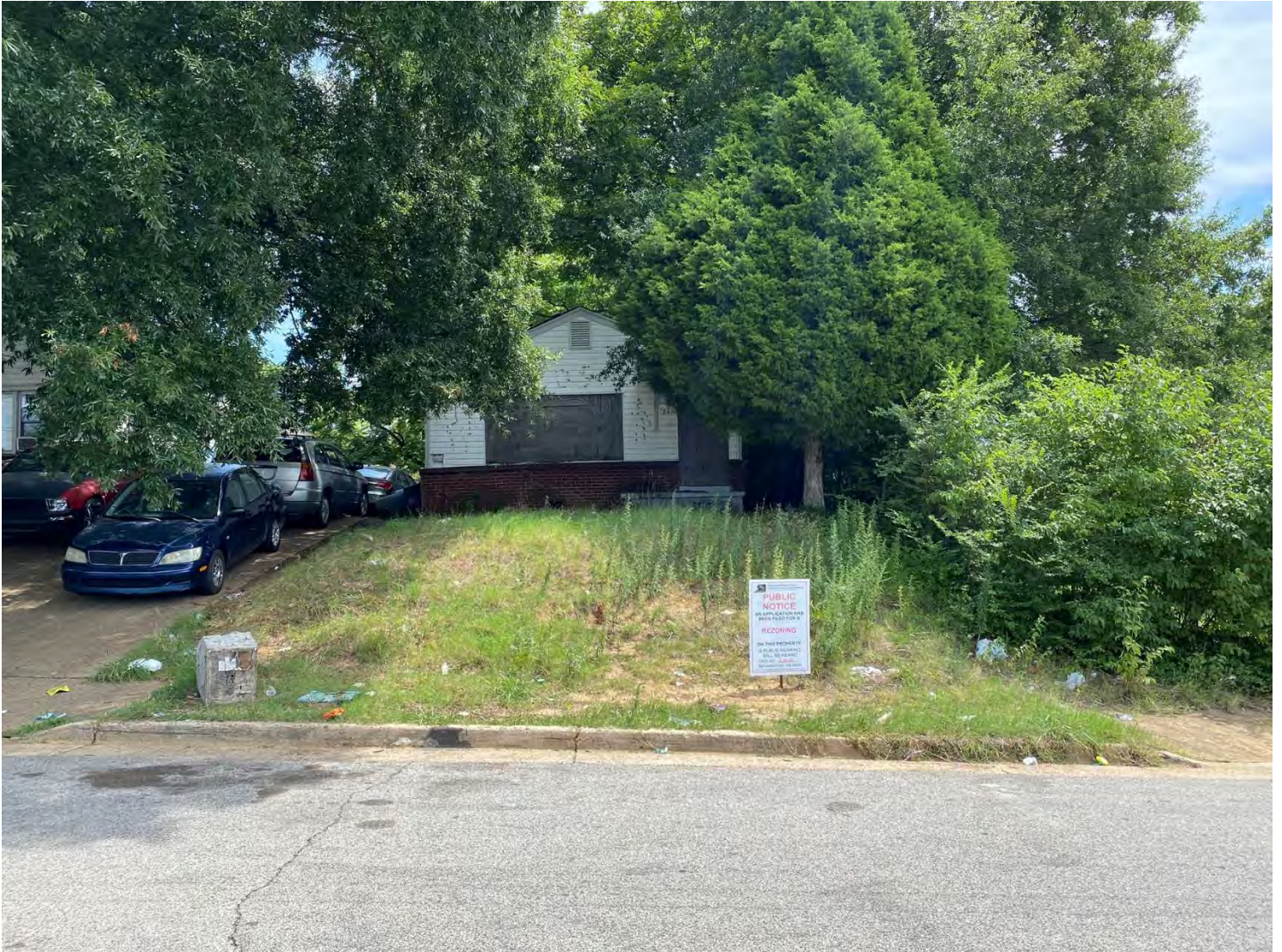
This subject structure – a vacant home – fronts Belt Line.
