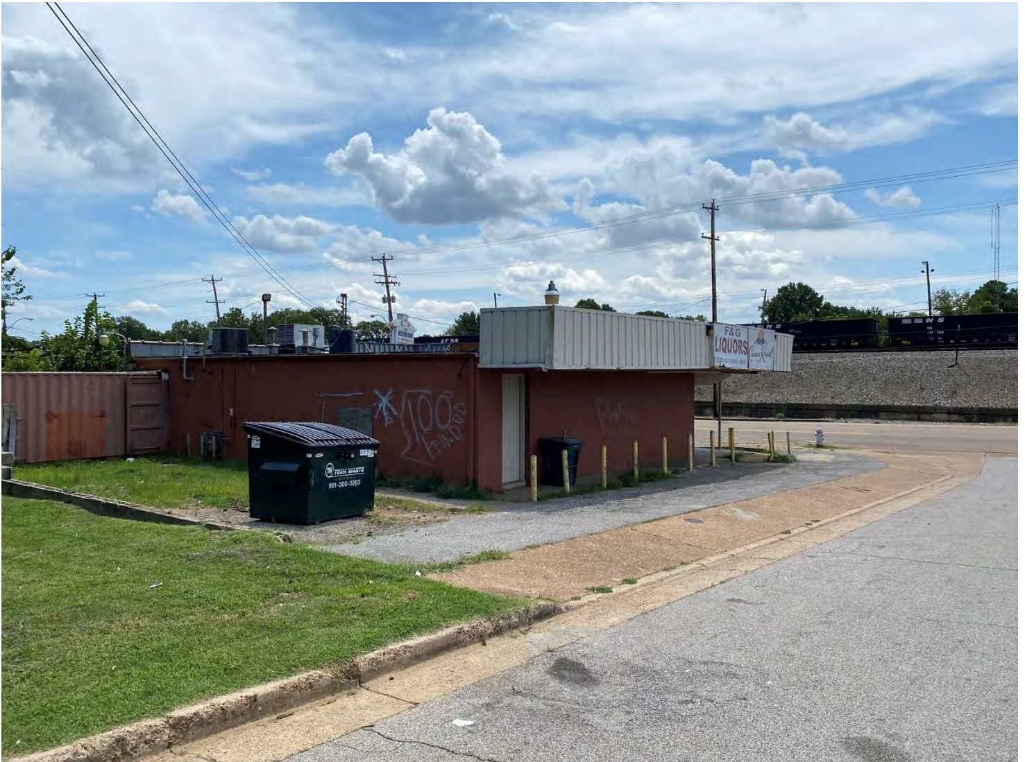
View of subject structure – a vacant liquor store – from Belt Line
