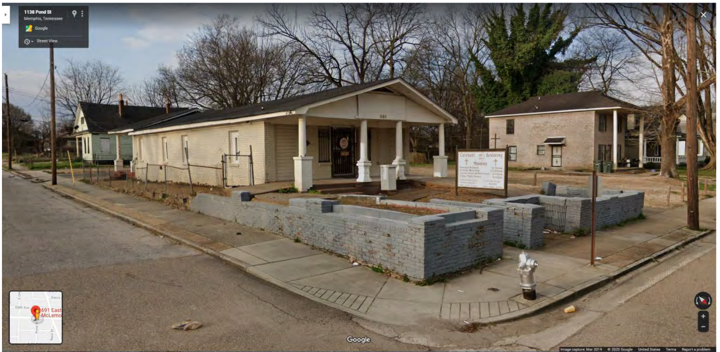
View of Covenant Restoring Ministries principal structure from the intersection of East McLemore Avenue and Pond Street looking southwest
